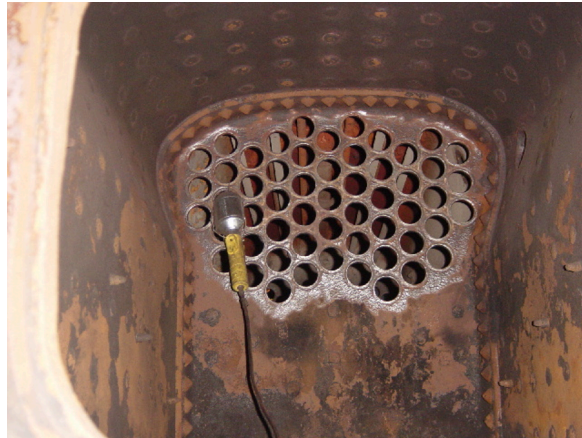
Fig. 6 Rear flue sheet.
