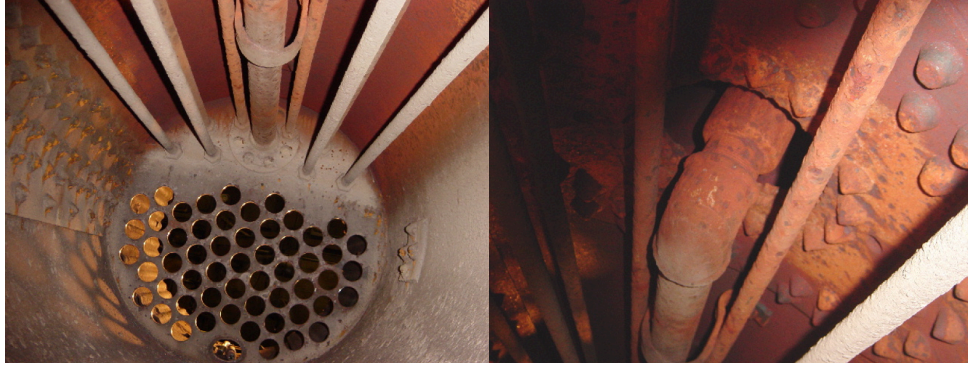
Fig. 7 Front flue sheet showing tube ends and internal features.
